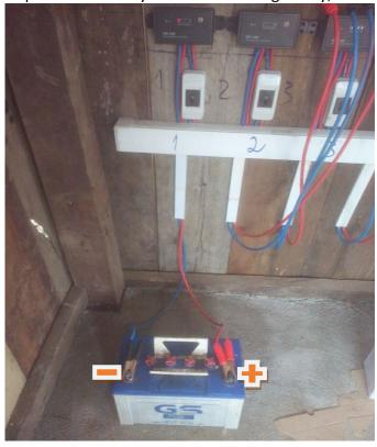
2. Read the light displayed on controller, make sure that there is percentage (%) light on the controller. If no light display, please check battery clamp or wire, maybe not connect properly. And if remain problem, please check wire connection again, and please contact technicians for assistance one the last page.
